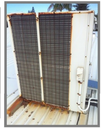
Actual instances of case corrosion which could have been prevented with a RetroMax
