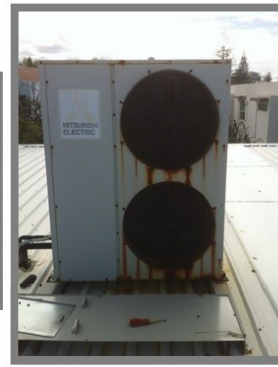
Actual instances of case corrosion which could have been prevented with a RetroMax
